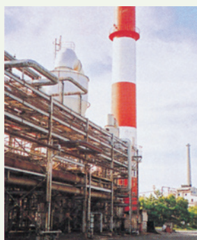
Desulfurization facilities attached to boilers at our Tokushima Plant
