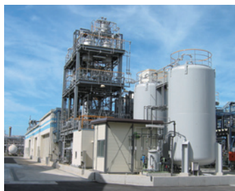
Tsurumi Soda Co., Ltd. plant
