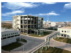
TOA-DIC Zhangjiagang Chemical
