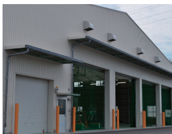
Tube container filling yard at the Tokushima Plant
