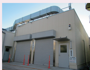
New analytical lab at the Yokohama Plant completed in 2019
