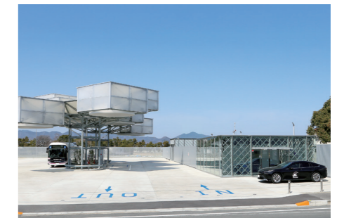
Toagosei Hydrogen Station Tokushima
