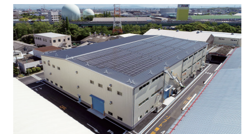
Nagoya Plant, Injection Plant No. 2 (completed in March 2021)
