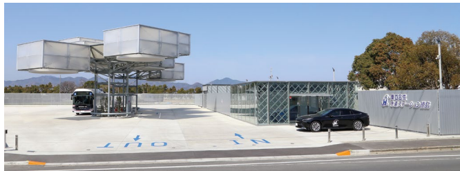
Toagosei Hydrogen Station Tokushima
